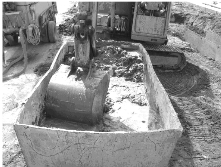
Figure 8. Soil-based flowable fill mixed with a backhoe
